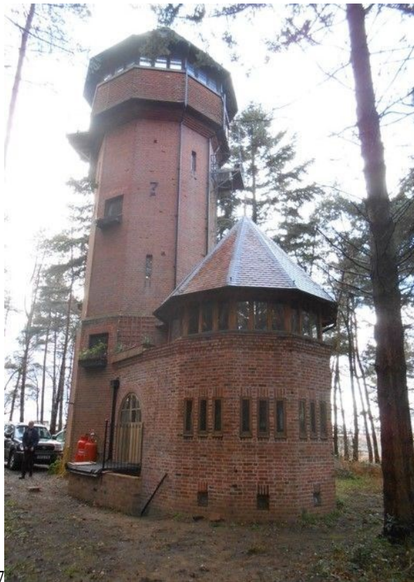
Geo. Cawston's Water Tower 1897
