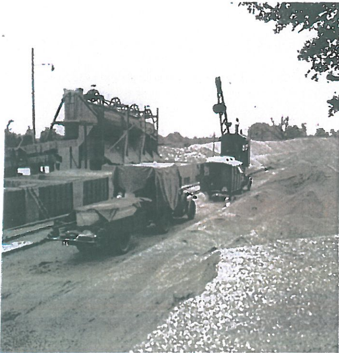
The column at the gravel-washing plant the next morning, with the Silver Eagle towing the 'old pattern of caravan' (an Eccles), and the Morris lorry to which was attached the trailer, on which lay the dinghy covered by a green cloth.
